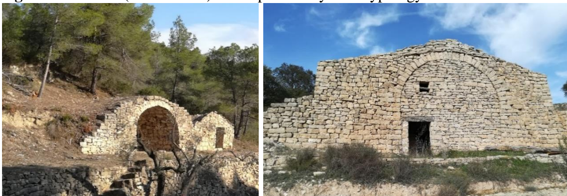
Figure 10. Cabins (La Fatarella). Examples of drystone typology located in la Fatarella.
