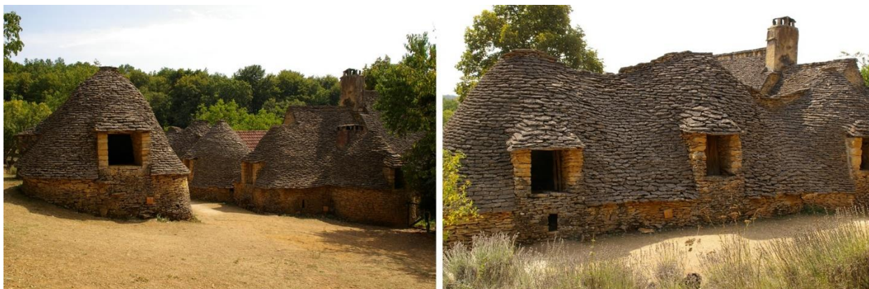
Figure 2. Les Cabanes de Breuil. On the left: view of a part of the cabins. On the right: triple cabin.
