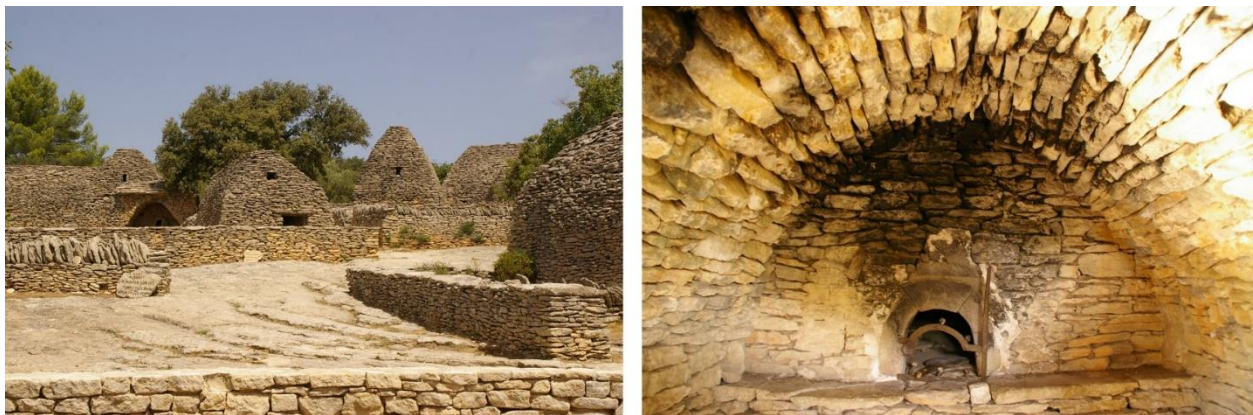
Figure 1. Drystone constructions in the village of Bories. On the left: view of a part of the village. On the right: inside view of a cabin.
