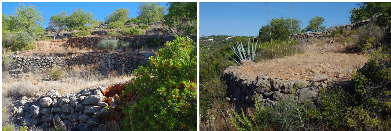
Figure 6. Cerro de São Miguel (Algarve). On the left: drystone walls and terraces. On the right: threshing floor made with a drystone wall.
